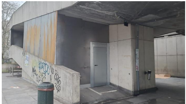
Figure 18. The barricaded ramp near the Cube.
